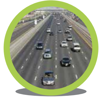
Six Lane Expressway
